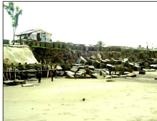
Fig. 2(b). Flood embankment behind the beach has failed under wave action
