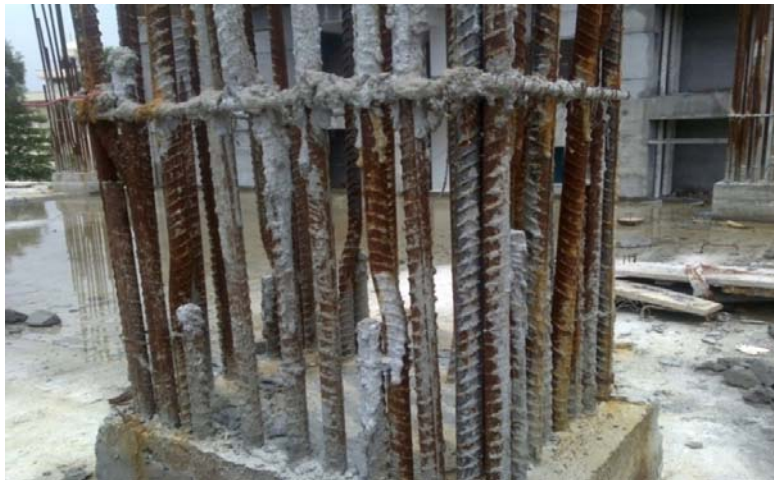
Fig.1. Lap splices in column
