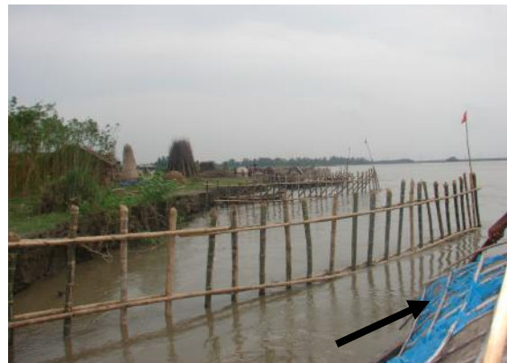
Fig. 4. Bamboo Bandals constructed in the Jamuna River ( Rahman et al. , Hydro conference 2009)
