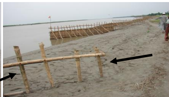
Fig. 5. Photographs showing bandals in 2009 flood and that of after flood
