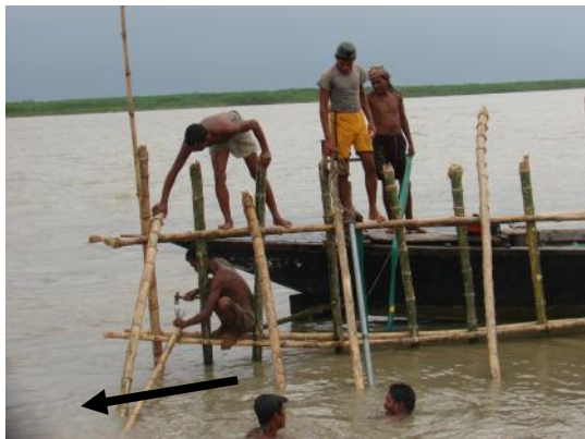
Fig. 4. Bamboo Bandals constructed in the Jamuna River ( Rahman et al. , Hydro conference 2009)
