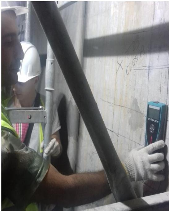
Fig. 5(a). Usage of Rebar Locator.
