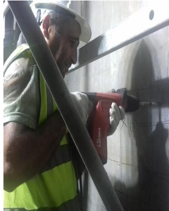
Fig. 5(b). Drilling of 48 mm hole for placing Anchor.
