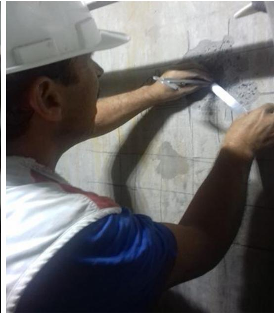
Fig. 9(b). Measuring the length of destruction.
