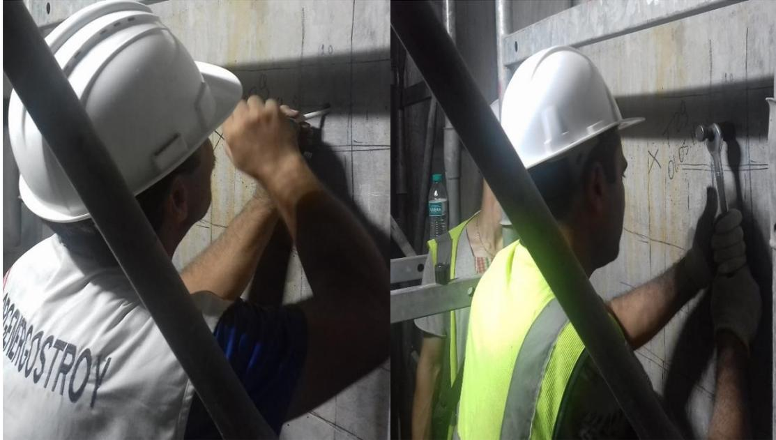
Fig. 6(a). Clearing dust from the hole.
